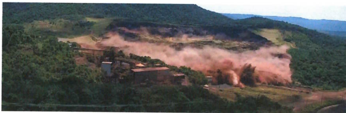
Figure 9. Failure of Feijão tailings dam I due to rapid flow liquefaction [10].
