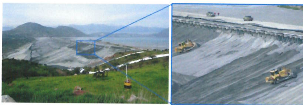
Figure 3. Las Tórtolas downstream sand dam [3]: (a) typical cross-section, and (b) flattening and compacting the downstream slope.
