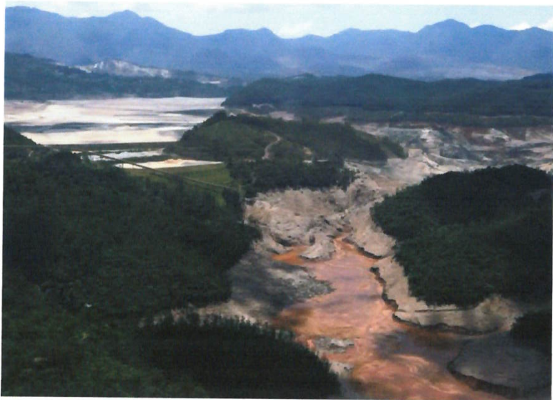
Figure 8. Failure of the Fundão tailings dam due to rapid flow liquefaction [9].
